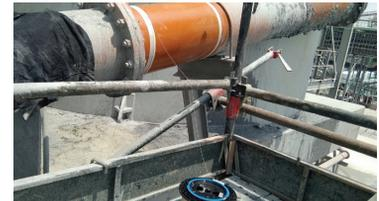
Silixa’s non-intrusive process metering technology enables flow distribution monitoring throughout an entire plant, mine or oilfield environment simply by using a single length of fibre-optic cable.
