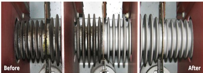
Electrical insulators should be inspected for evidence of physical damage or contaminated surfaces. Damage caused by electrical distress is normally evident on the surface of insulating members in the form of corona erosion or markings or tracking paths.
