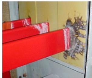
Electrical discharges might also form around bolt heads or other sharp projections that are not properly insulated or shielded.
