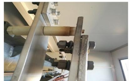
Loose core clamping (bolts) system can lead to high temperatures that can lead to premature failure.
