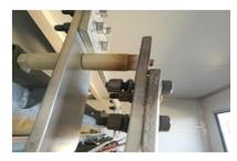
Loose core clamping (bolts) system can lead to high temperatures that can lead to premature failure.
