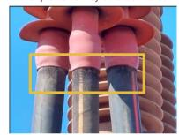
Water ingress in the cable causes neutral or shield corrosion and water tree development, eventually leading to premature cable insulation failure.
