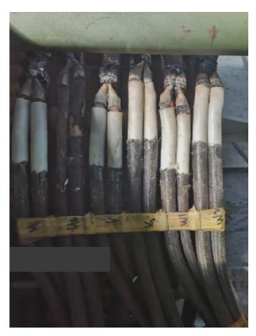
The Siwo-Kul cables are part of the MV motor power circuit and if any of these fail, the motor will be out of service for a long time due to contamination and other factors.
